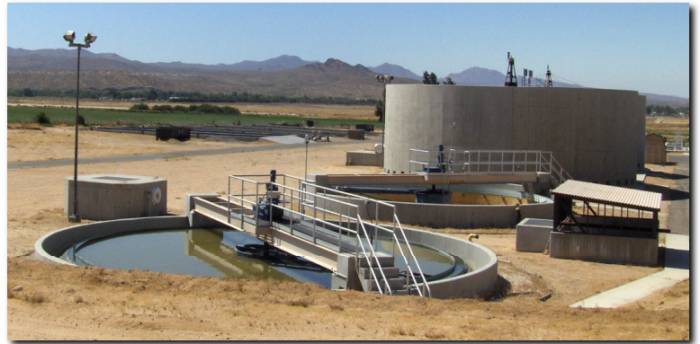
Above: Trickling Filters process wastewater utilizing a media with a biological mass. Below: View of primary clarifiers and trickling filter.
