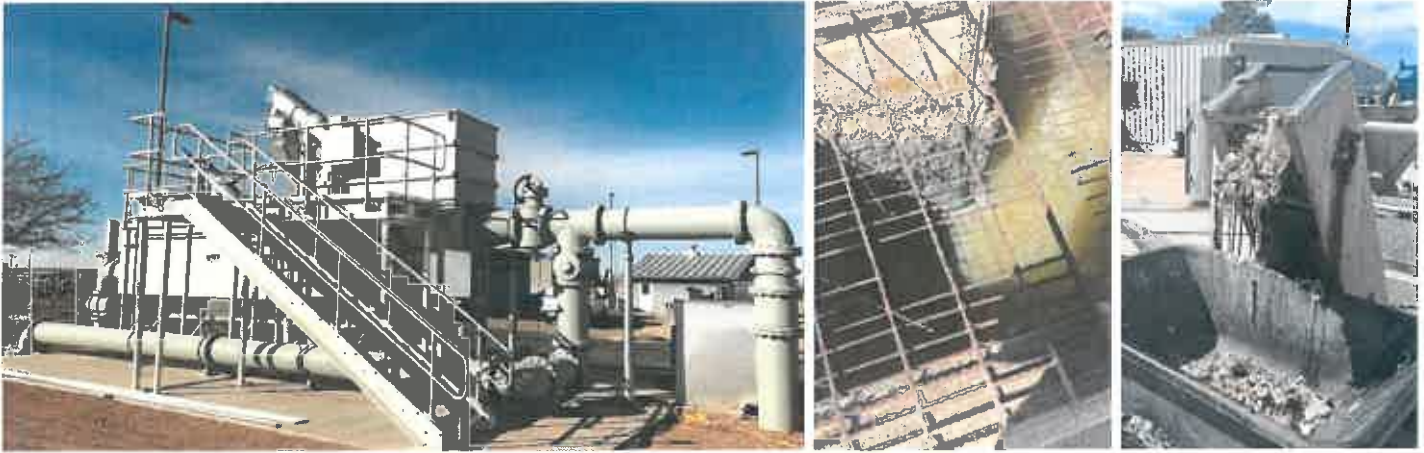
▲ Left to Right Example of Packaged Headworks System with 6 mm Fine Screen and Aerated Grit.
